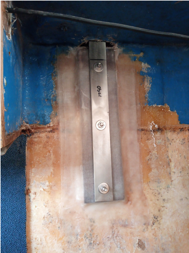
Chainplate for upped shroud installed
