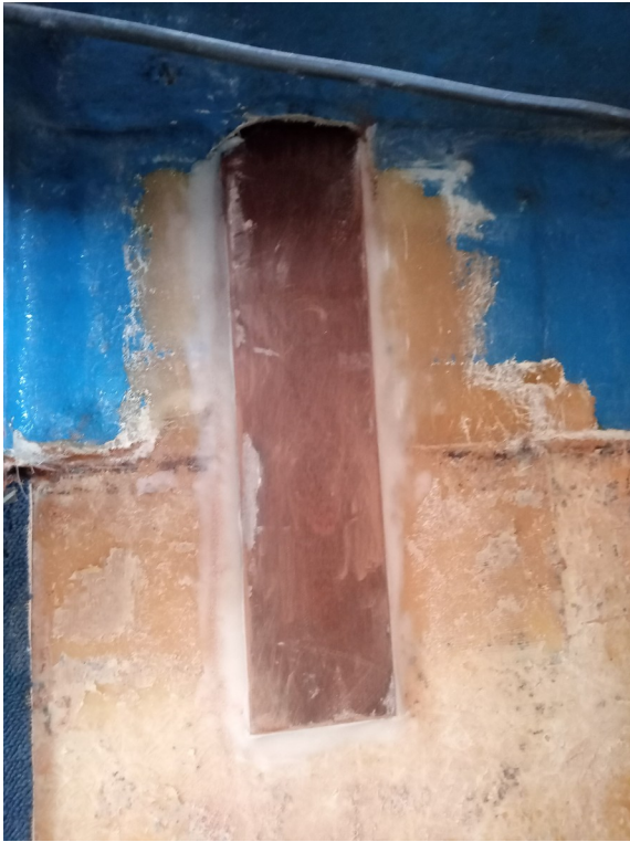
New plywood backing plate glued in (upper shroud)
