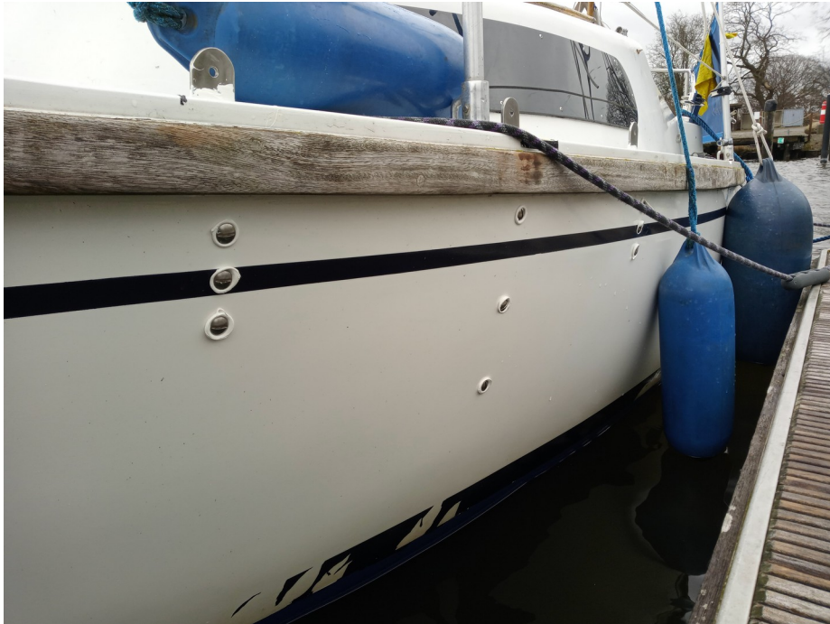
Bolt heads showing the chainplate attachment.
