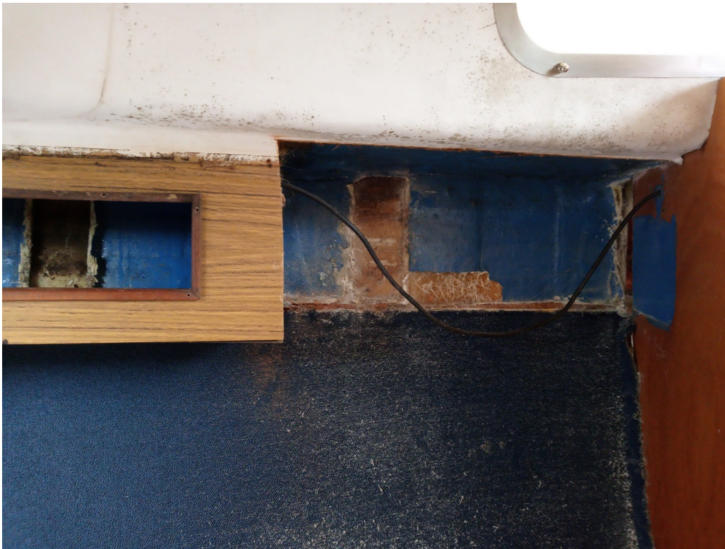
After removal of the chainplates (and a cupboard)
