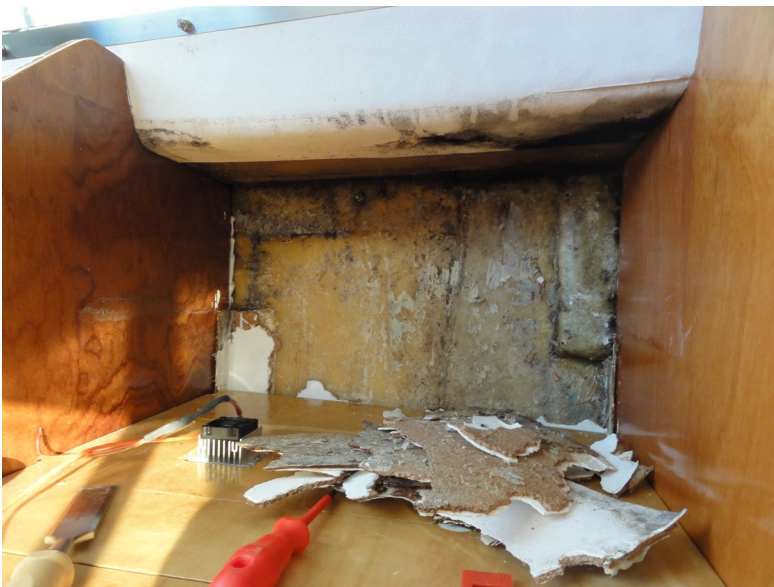
Chainplate pocket visible next to bulkhead on the right in the galley area after removal of cupboard and insulation
