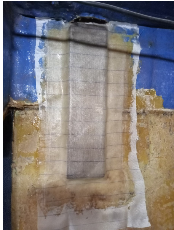
Glassed over and covered in peel ply
